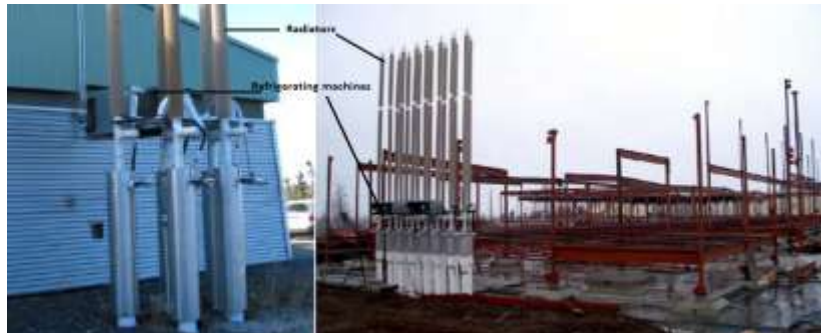
Fig. 11 Hybrid thermosyphon installation in Inuvik hospital (Modified after Holubec 2008).
