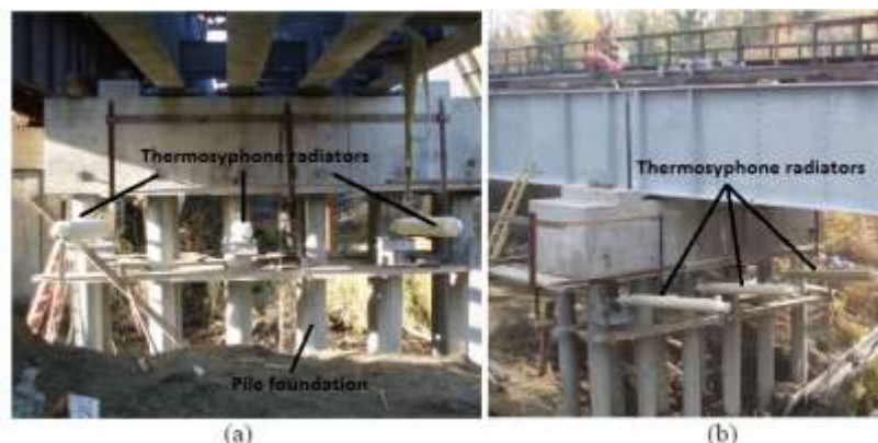
Fig.17 Thermosyphone condenser installation on bridge pier piles (a: courtesy of Arctic Foundations Inc, and b: courtesy of Alaska Railroad Corporation's)(Modified after Krzewinski and Ross 2013).
