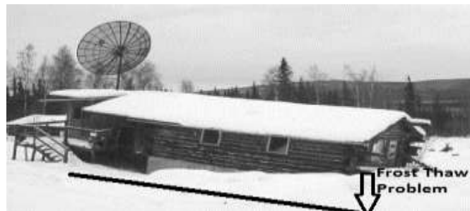
Fig. 1 Large differential settlement in a structure in permafrost region, Fairbanks(Modified after Clarke, 2004).
