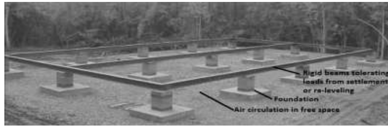
Fig. 3 An example of pad and post system (Modified after Clarke, 2004).
