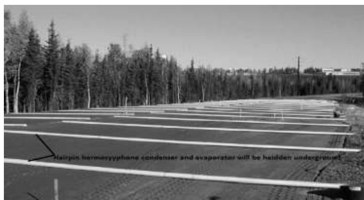
Fig. 14 Hairpin thermosyphon condensers used in Thompson drive, Alaska (Modified after Xu and Goering 2008).
